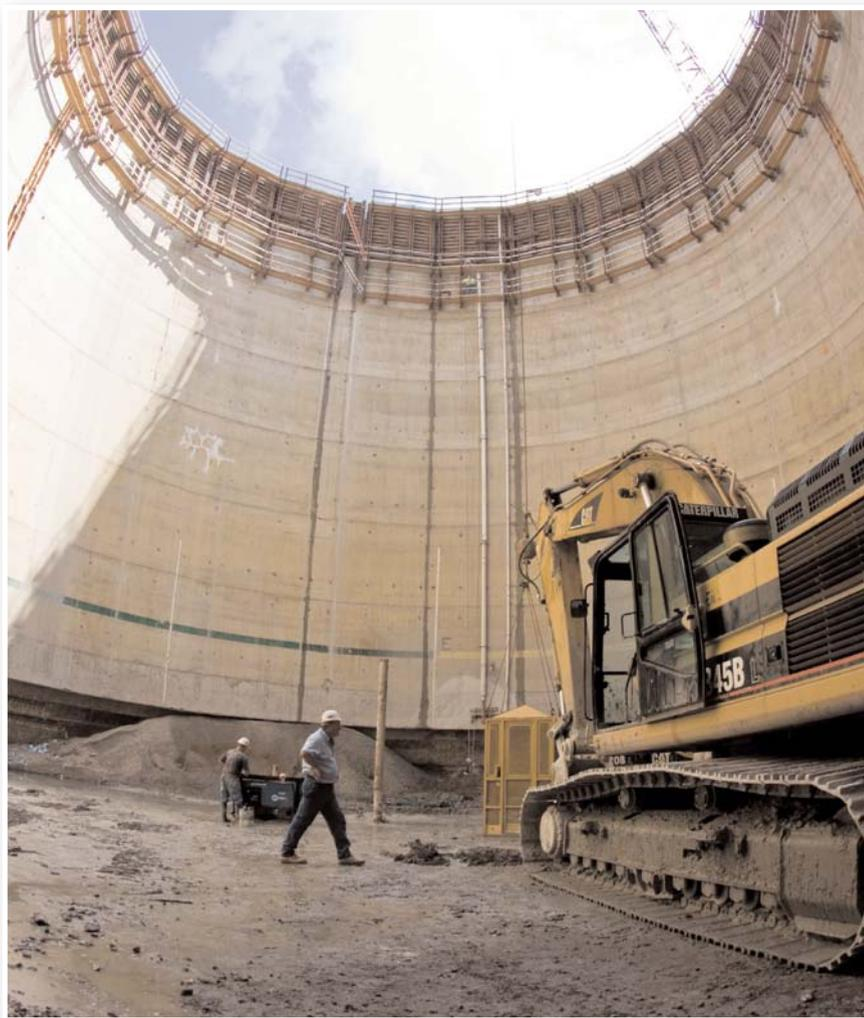
*The treatment shafts are constructed using the sinking caisson construction method.*
