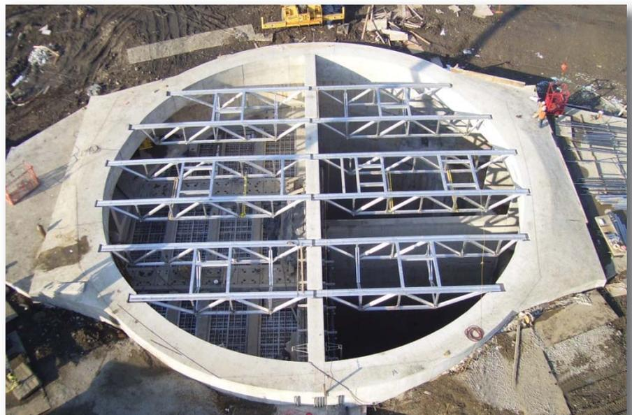
Figure 2. If disinfection is not required, the design still provides capture volume, skimming, settling and screening, all within a compact footprint.
