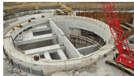
Applied Engineering Technologies' "treatment shaft technology" stores and treats floods of wastewater from combined sanitary and storm sewers.
